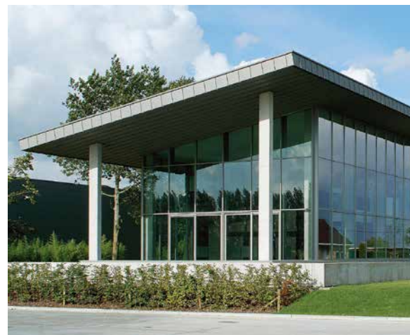
The UNILIN, division insulation headquarters
