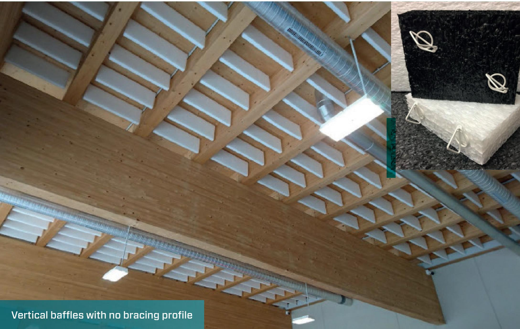
Vertical baffles with no bracing profile
