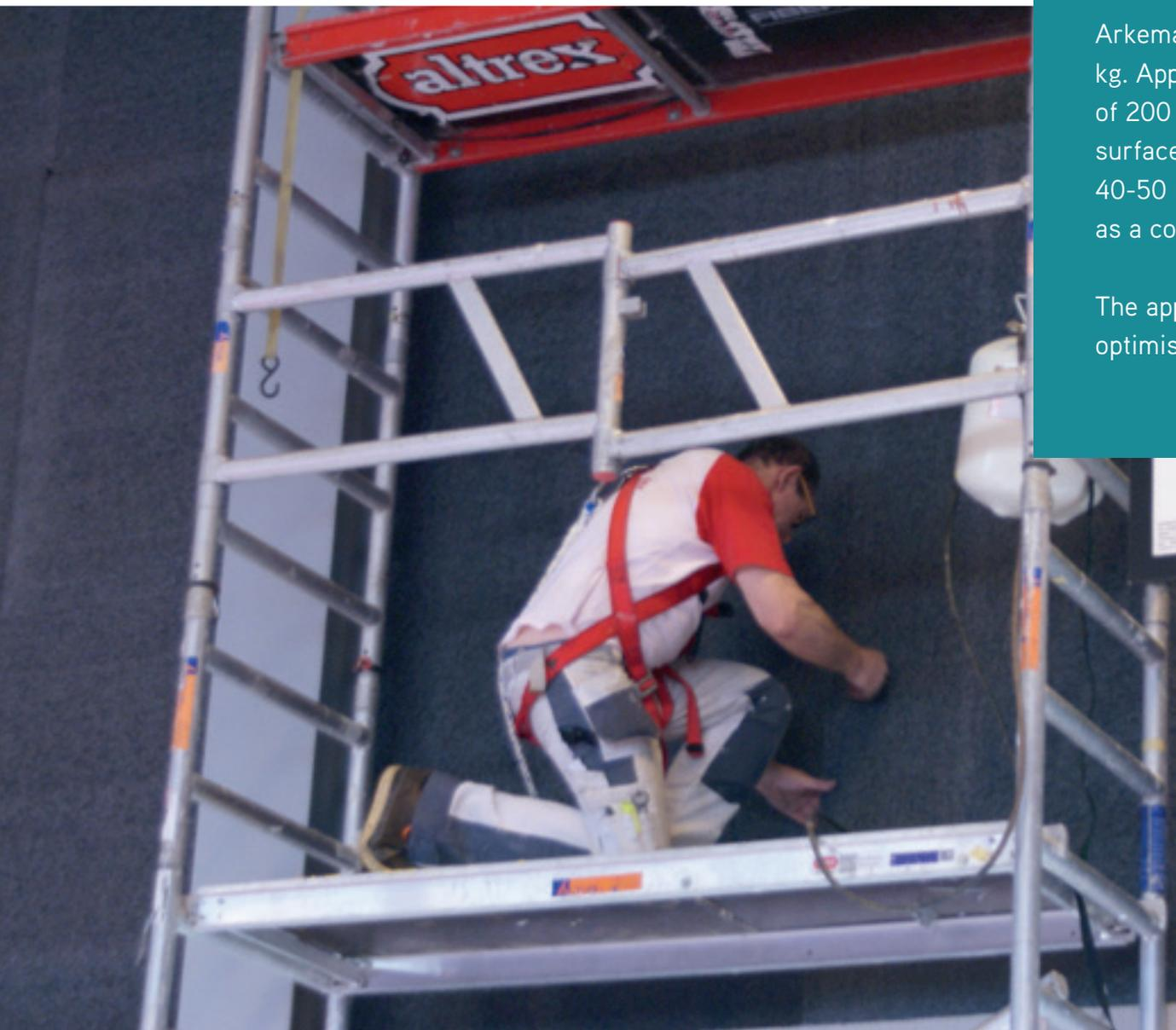
Arkema Cofix S is supplied in a canister of 25lt or about 20 kg. Apply Cofix S to both corresponding surfaces at a rate of 200 grams per square metre. Adhesive may be applied to surfaces with spray gun or brush. This is sufficient to cover 40-50 m<sup>2</sup> of coverage by applying it on both bonding faces as a contact adhesive.
