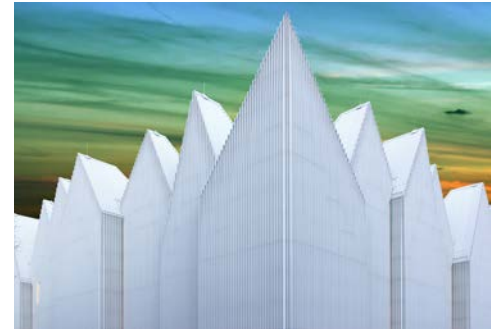
Szczecin Philarmonic (Poland) – Arch. Studio: Barozzi Veiga
