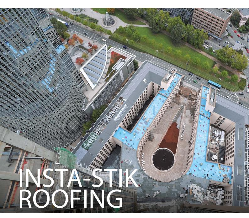
Adhesive for insulating and waterproofing flat roofs.
